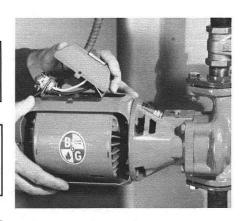
The conduit box cover must be removed and all electrical wires must be disconnected prior to separating the motor from the bearing assembly. The photograph illustrates the removal of the conduit box cover. This procedure is followed by the removal of the wire nuts and the flexible conduit connector.
