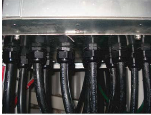
Illustration 5.16: Example of proper installation of the gland plate.
